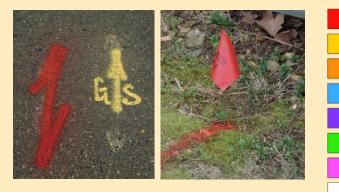
Electric power lines Gas, oil, or steam pipelines Communications lines, cables, or conduit Potable water Reclaimed water, irrigation, and slurry lines Sewers and drain lines Temporary survey markings Proposed excavation
