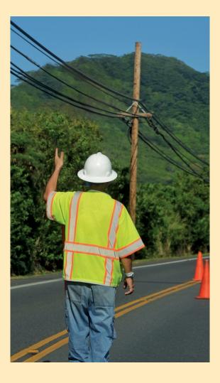
For Tools and Equipment Other than Cranes and Derricks Used in Construction, Observe the 10-Foot Rule
